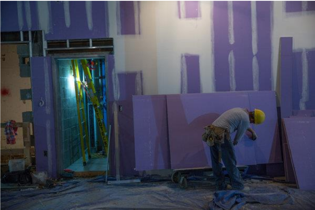
The renovation in progress.
